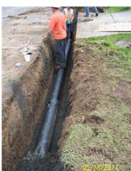
• The Glen Avenue Waite Street waterline has been replaced with a new 8" cast iron pipe.
