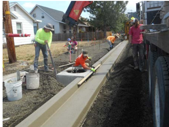
2768 – Slip formed curb/gutter East end Rt. Side 2770 – Setting CG-3 inlet top
