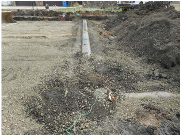
2772 – 12-inch storm sewer cross pipe at Sta. 11+06
