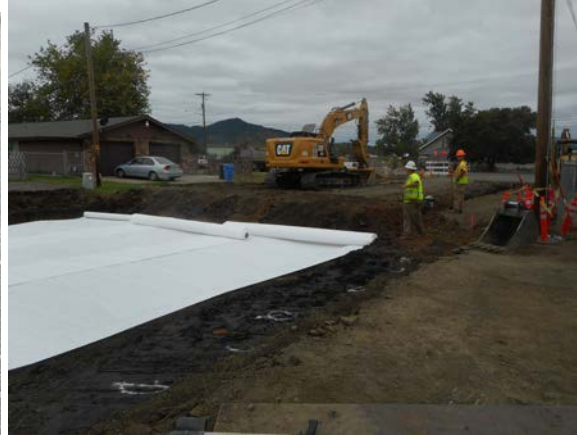
2766 – End of day excavation progress
