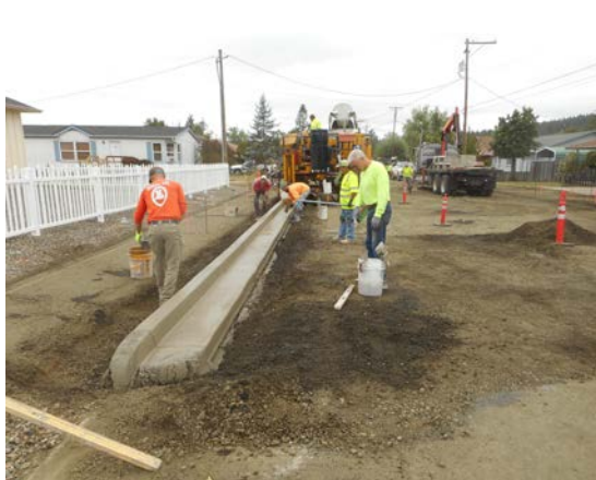
2768 – Slip formed curb/gutter East end Rt. Side 2770 – Setting CG-3 inlet top
