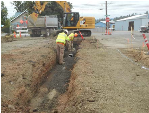
2767 – 12-inch storm sewer, looking westerly
