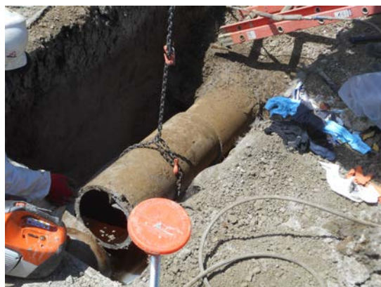
2712-East End – Removing Transite section
