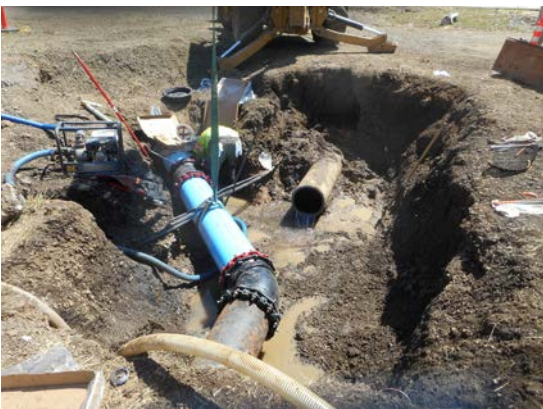
2696-West End – New connection in place
