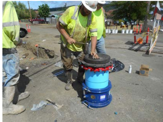
2686- East End – Building temp. cap connection
