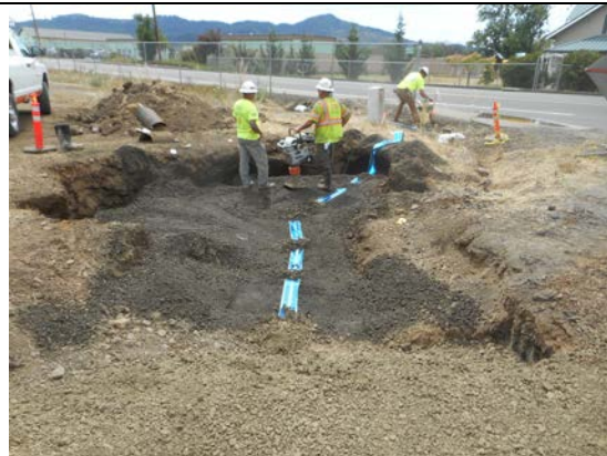
2721-West End – Backfilling & marking WL
