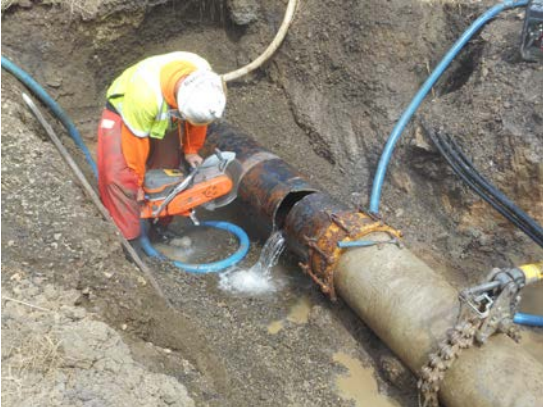
2682 – West End – Opening steel pipe to drain
