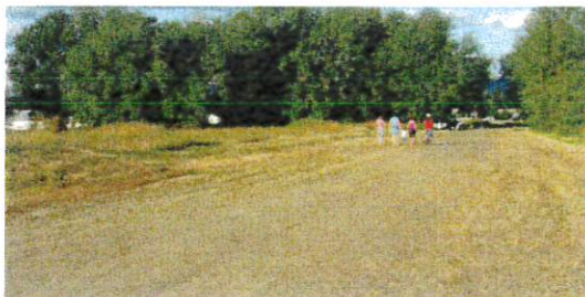
Red Rock Road capped with gravel in Sutherlin
