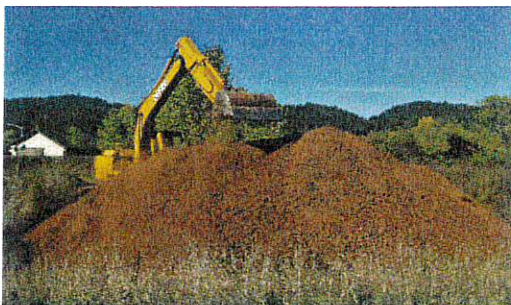
Stockpiling Red Rock Road soils for landfill disposal
